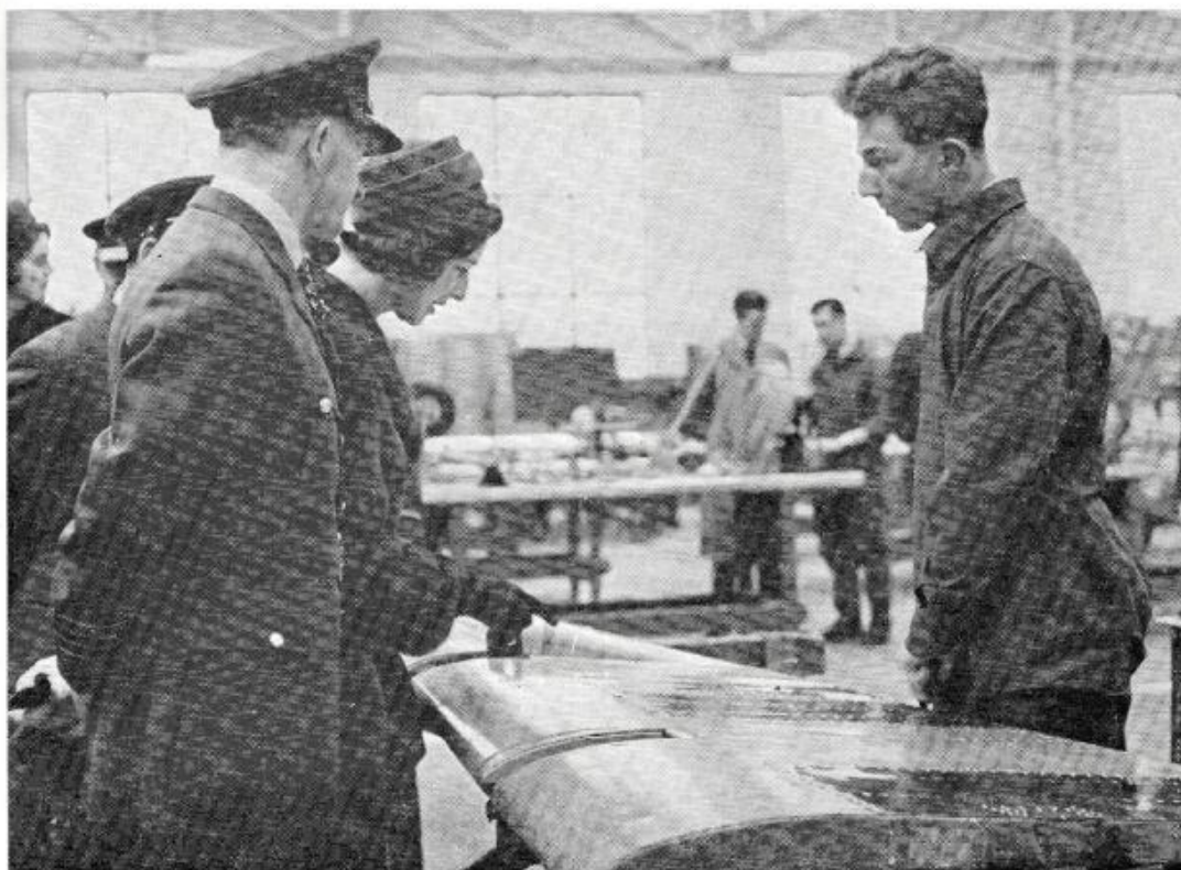
Corporal Aircraft Apprentice Smith of 102nd Entry, using a P.G.O. 3 pneumatic rivetting gun, demonstrates how a flush repair patch is inserted in a Javelin aileron.
